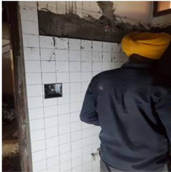
Restoration of Court Room No.8 is in progress
